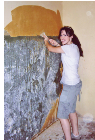
Above: Sami Matthews working on the renovation project.
